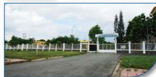
Water supply factory
